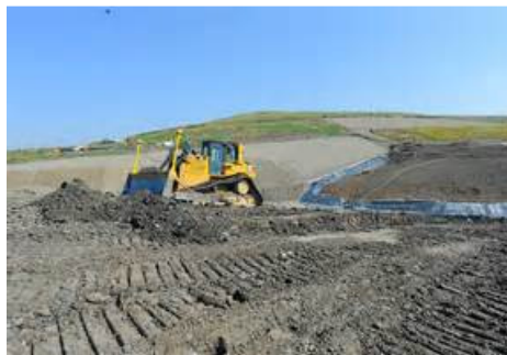
LAND FARM – CONTAMINATED SOILS
